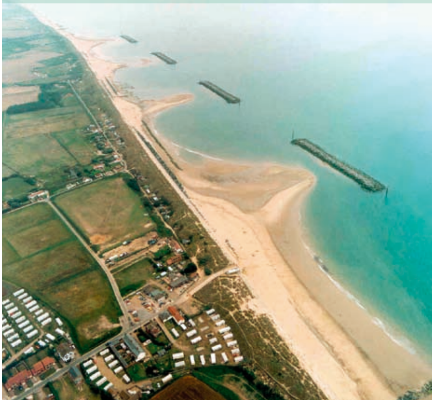
Sea Palling in Norfolk showing the breakwaters built to protect the coastline.
